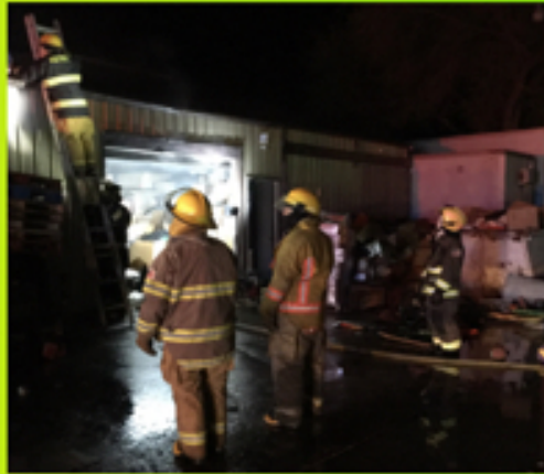
Building was a total loss
